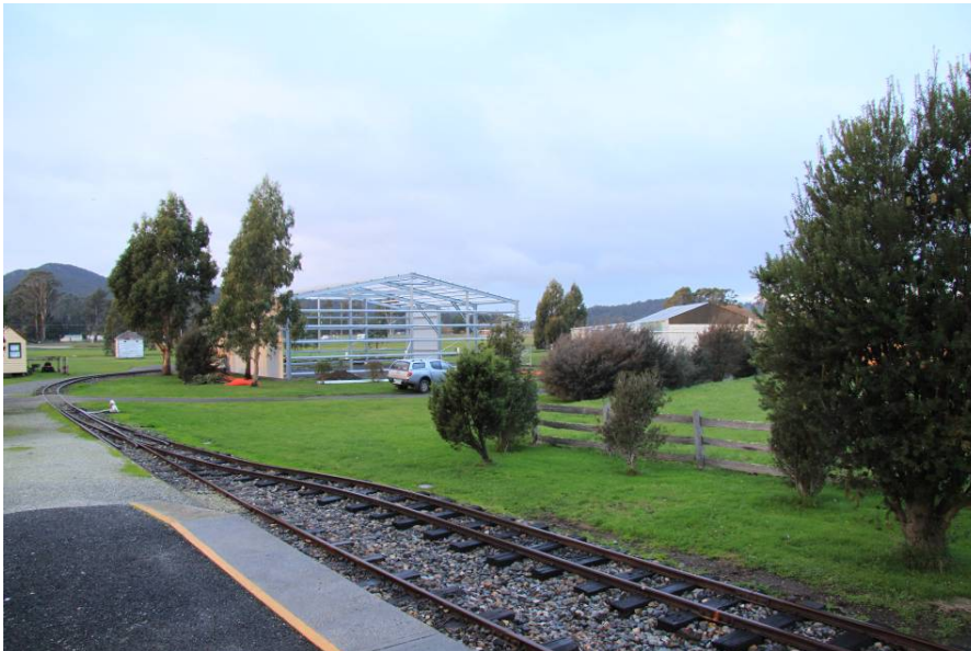
Caption: The new shed viewed from the Sheffield Railway Station platform.
